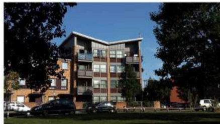
02. End block of apartments, Johnson Rd
