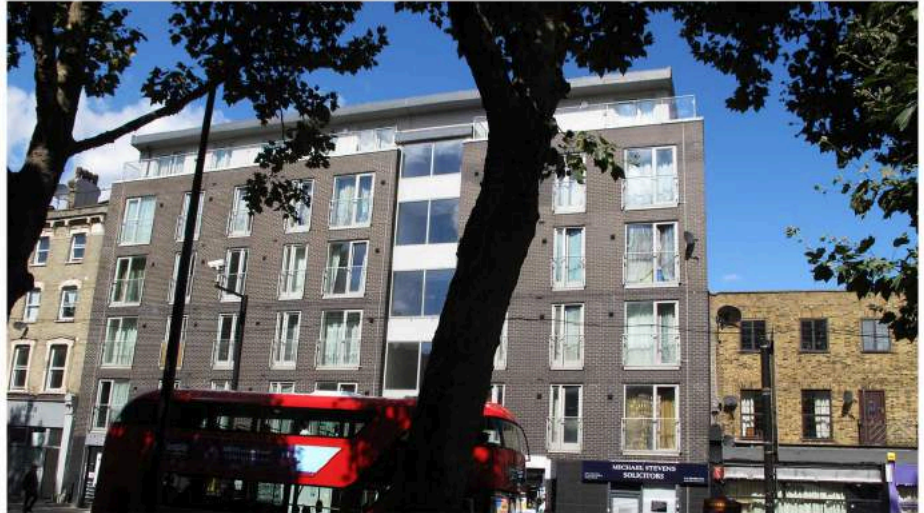
01. Photograph of the front facade facing New Cross Road
