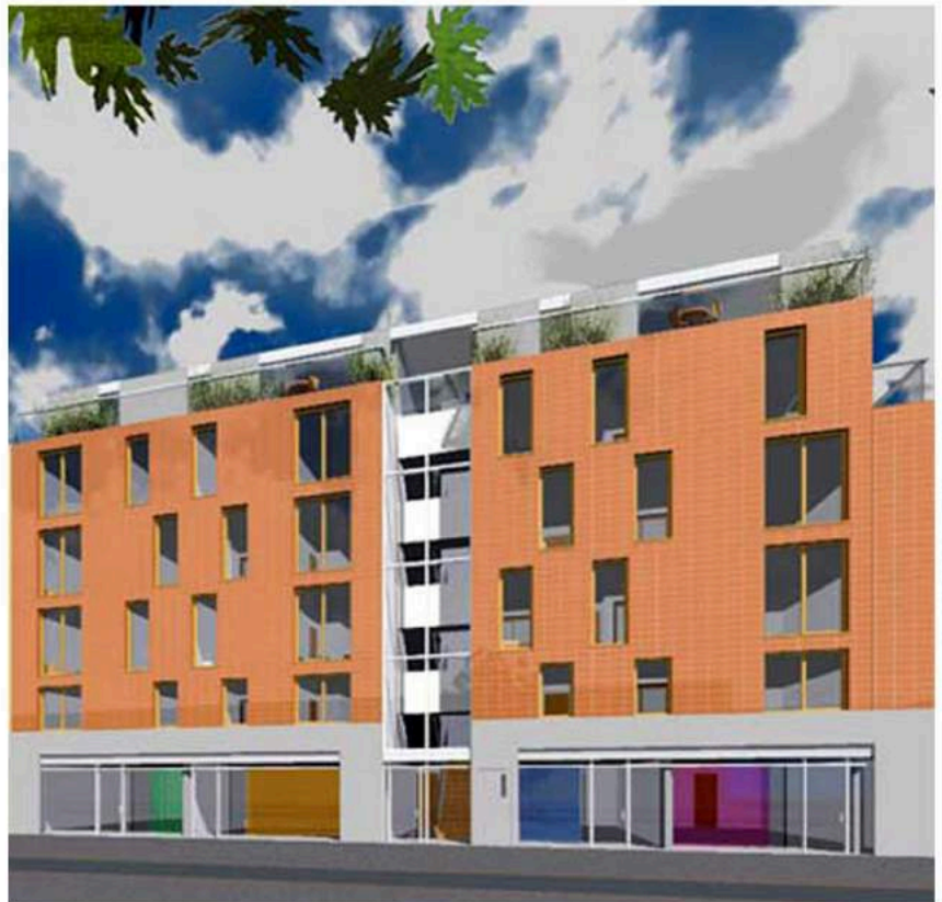
05. cgi of planning -approved front facade, with red terracotta tiles and coloured glazing
