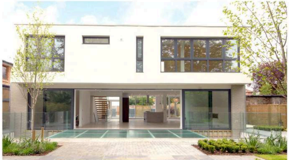
01. Photograph of rear elevation from the garden
