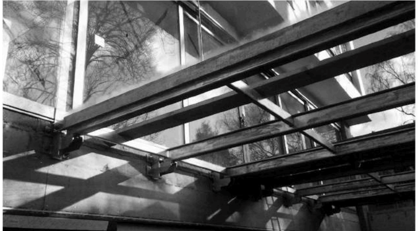
05. Construction of glass bridge over pool void
